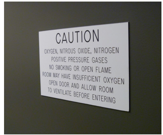
Figure 19. Equipment Room Wall Plate.
