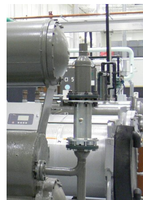
Figure 18. Rupture Disc.
